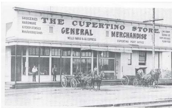
By 1904, the Cupertino Store Inc., located at The Crossroads where the Gulf Station is today, became the largest general store in the Valley, east of San Jose. Note the Interurban railway tracks in the foreground. Courtesy of Florence Deacon
