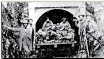
The Main Tunnel opened in 1847 at the head of Deep Gulch. Sherman Day, engineer and superintendent, stands at right.
