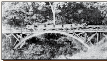
A donkey pulled the empty ore carts across the trestle over Deep Gulch to the reduction site.
