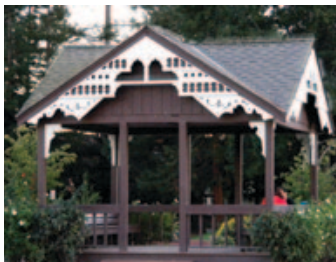
Gazebo Trim Mary & Stevens Creek Blvd. – Memorial Parkf
