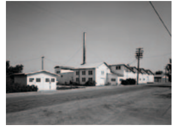
Woelffel Cannery 10120 Imperial Avenue – demolished
