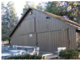
Glendenning Barn 10955 N Tantau Avenue – Hewlett Packard
