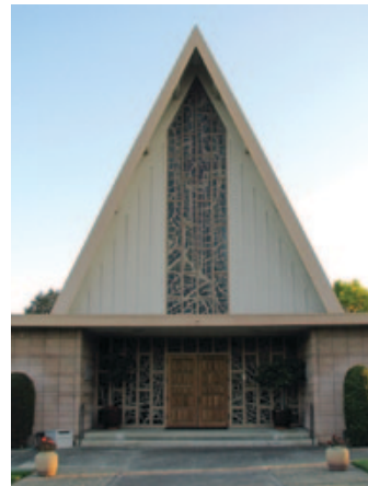
Union Church of Cupertino 20900 Stevens Creek Boulevard
