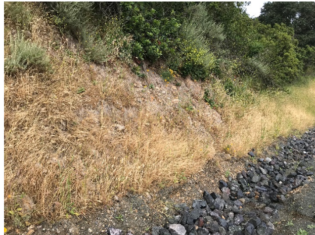
Figure 5 Road Cut at Cross-Section C-C'
