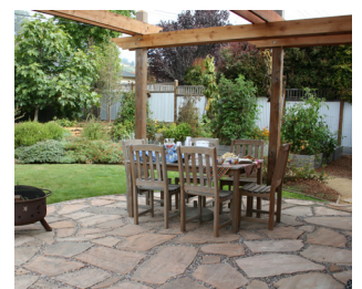
Flagstone with permeable joints
