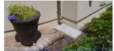
Splash block directs water to landscaping.
