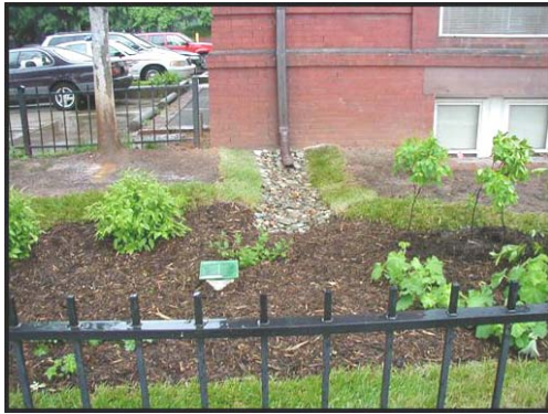
A Low-Impact Development Disconnected Downspout
