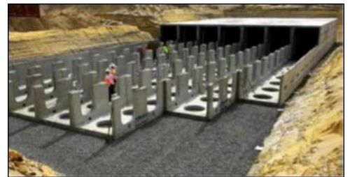
Figure 2-9 Subsurface vault, under construction (Source: Conteches.com)
