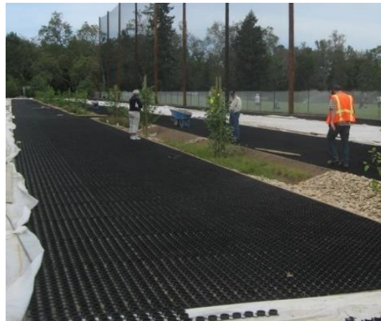
Figure 2-10 Completed green parking bays (above left) and parking bays under construction, showing the recycled plastic geocells that support vehicle weight (above right). (Source: City of Cupertino)
