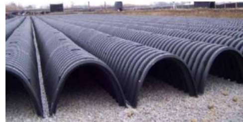
Figure 2-6 Subsurface infiltration system (Source: Conteches.com)
