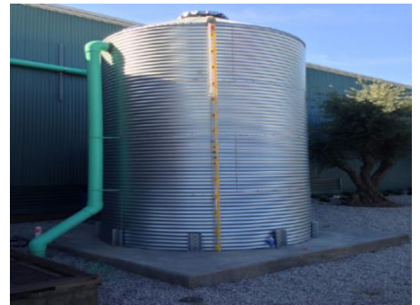
Figure 2-8 Rainwater harvesting cistern, Environmental Innovation Center, San José (Source: City of San Jose)
