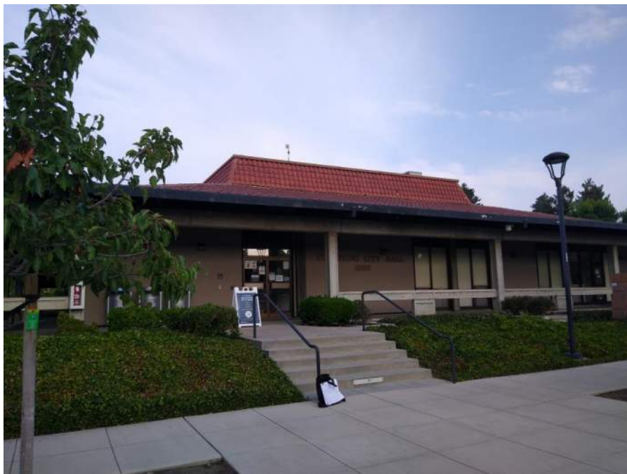
Photo e East Elevation
