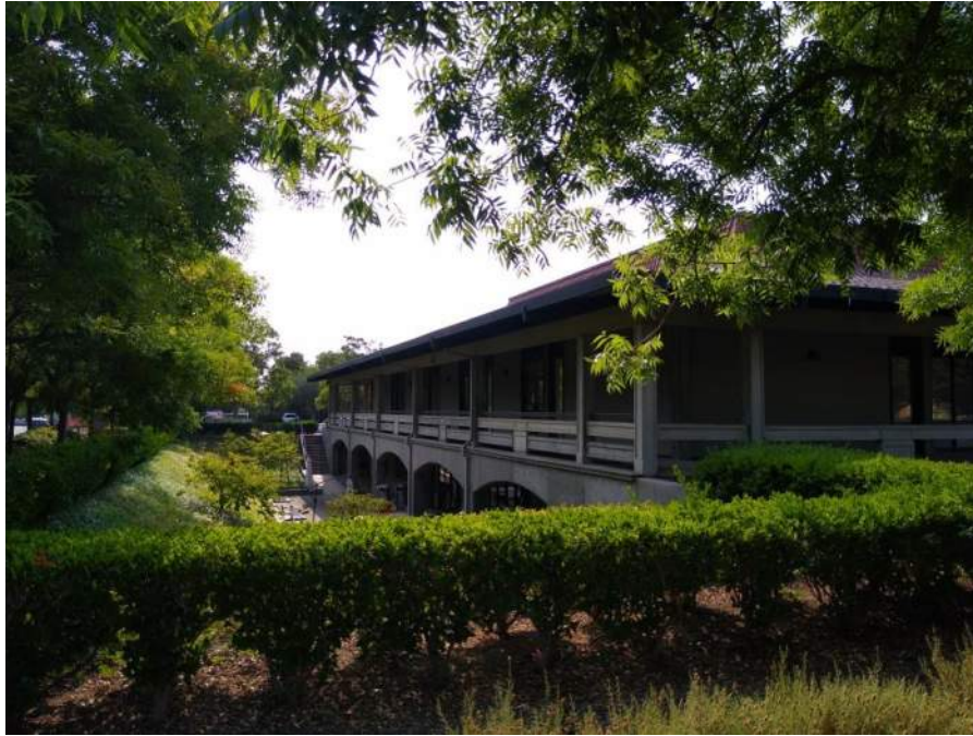
Photo 1 North Elevation with Elevated Veranda Slab
