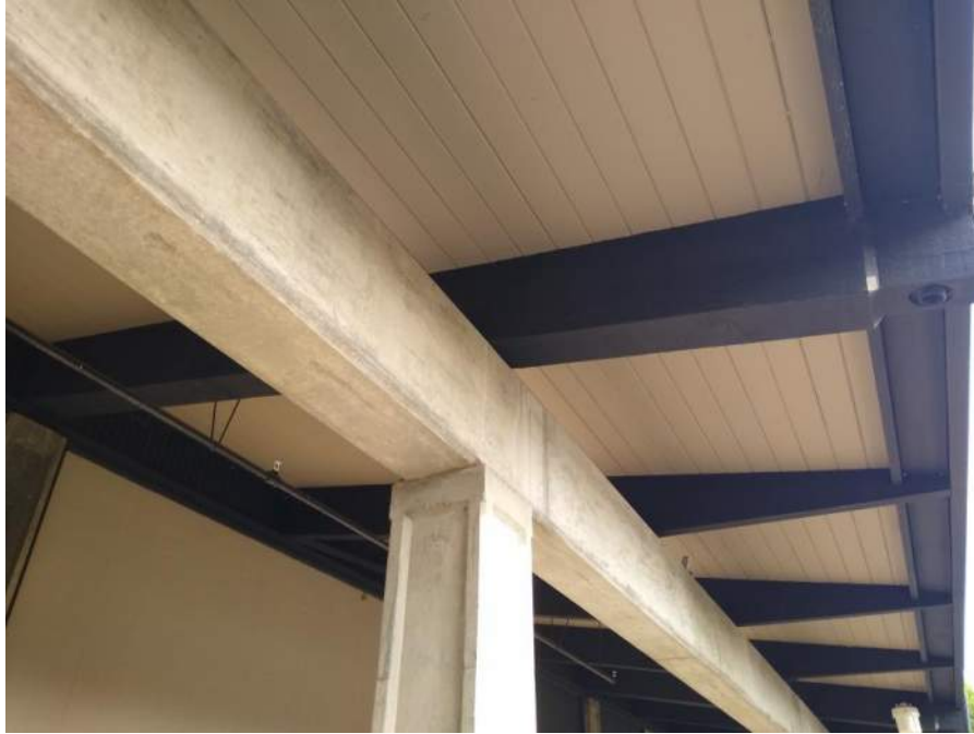
Photo 2 Veranda Concrete Beam
