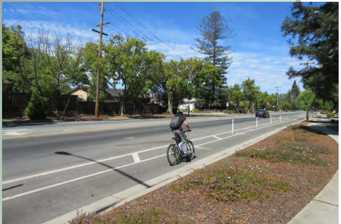
Site Photo 8: Buffered bike lanes on both sides of Stelling Road are popular with cyclists.
