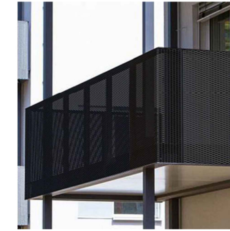
STEEL RAILINGS, W/ PERFORATED PANEL PAINTED
