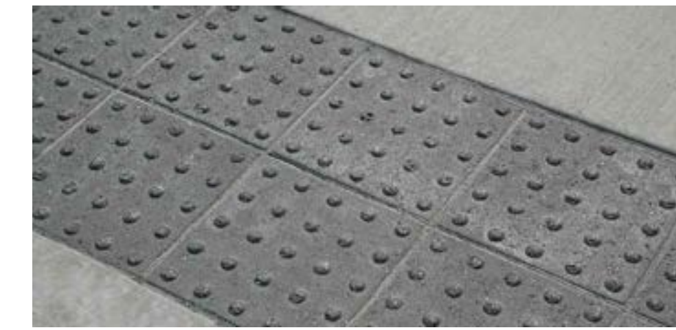
4 TRUNCATED DOMES (ON SITE) N.T.S. PHOTO
