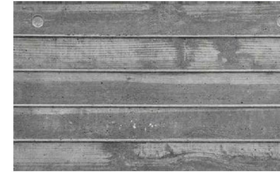
5 BOARD FORM FINISH CONCRETE N.T.S. PHOTO
